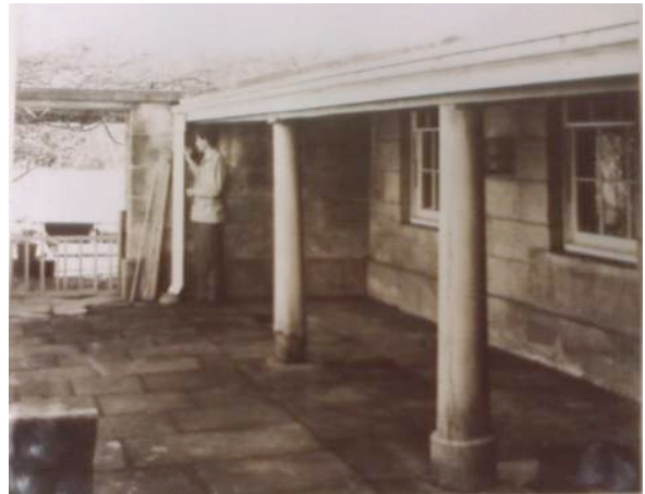
Figure 32: North side of internal courtyard
