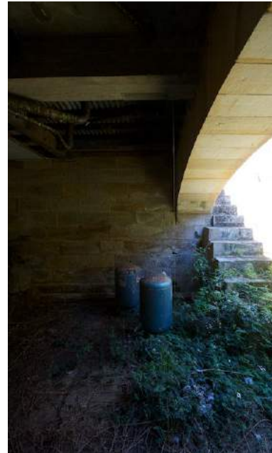
Figure 132: External stair and stone archway to basement, looking west. Paul Davies 2013.
