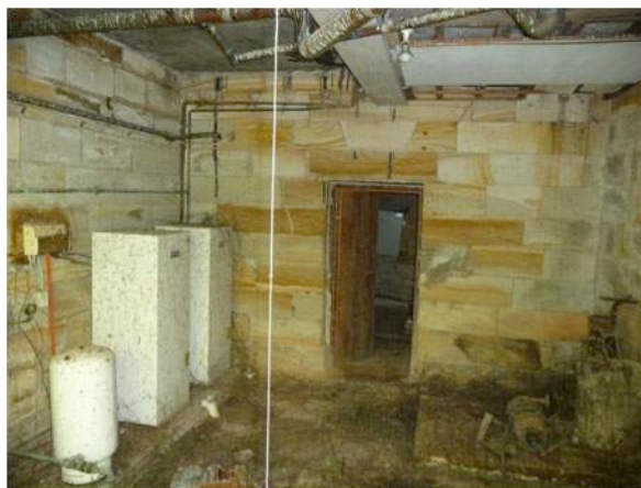
Figure 146: B12 open room accessed via external stairs off north wing
