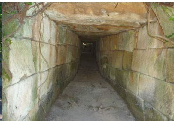
Figure 171: Sandstone drain under southern bridge. Paul Davies 2005.
