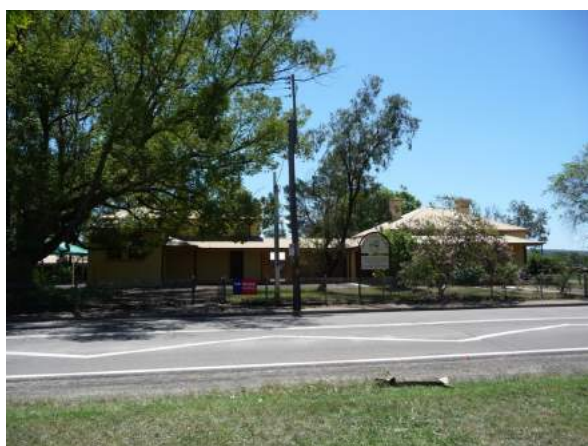
Figure 280: Mulgoa Public School, Mulgoa Road, looking north-west
