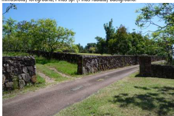
Figure 204: Perimeter stone wall around Sorensen's garden, added by current owner in early 1980s, looking north. Paul Davies 2014.
