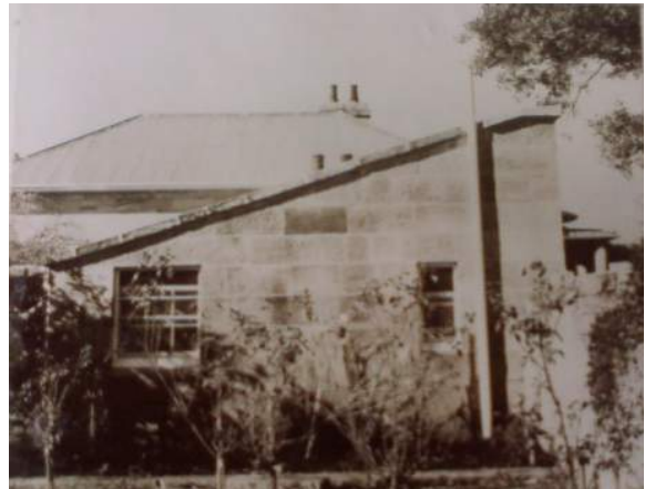
Figure 26: West elevation of the separate cess pit structure (now removed)
