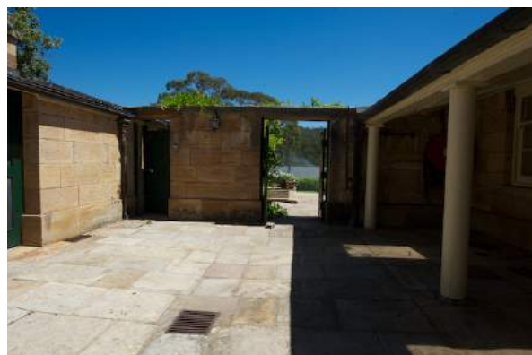
Figure 134: Internal courtyard, looking west. Paul Davies 2013.
