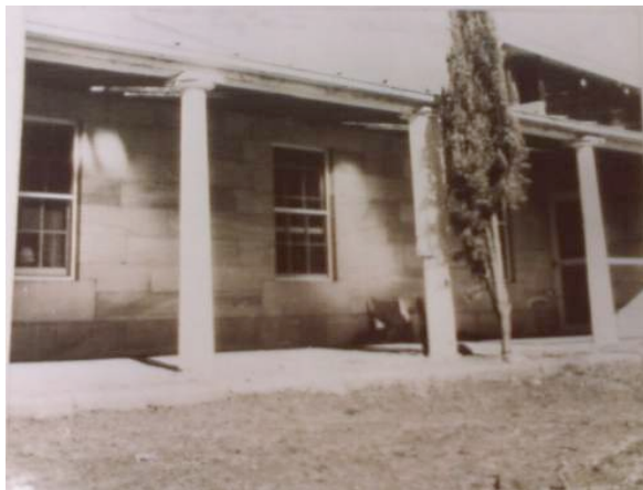
Figure 29: Verandah on north elevation
