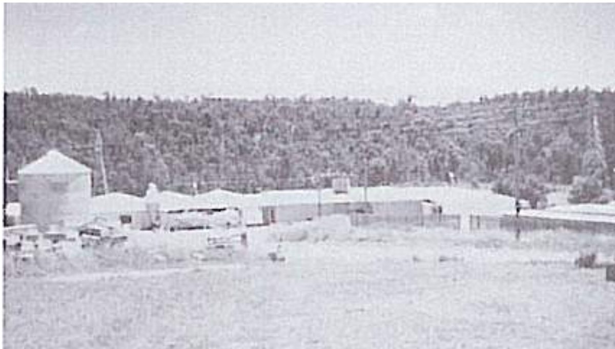
Figure 46: Chicken hatchery at Fernhill, c.1961. This building and the associated feed stores were erected for John Darling in the late 1950s; they have since been demolished and the area was redeveloped; Source: Private Collection
