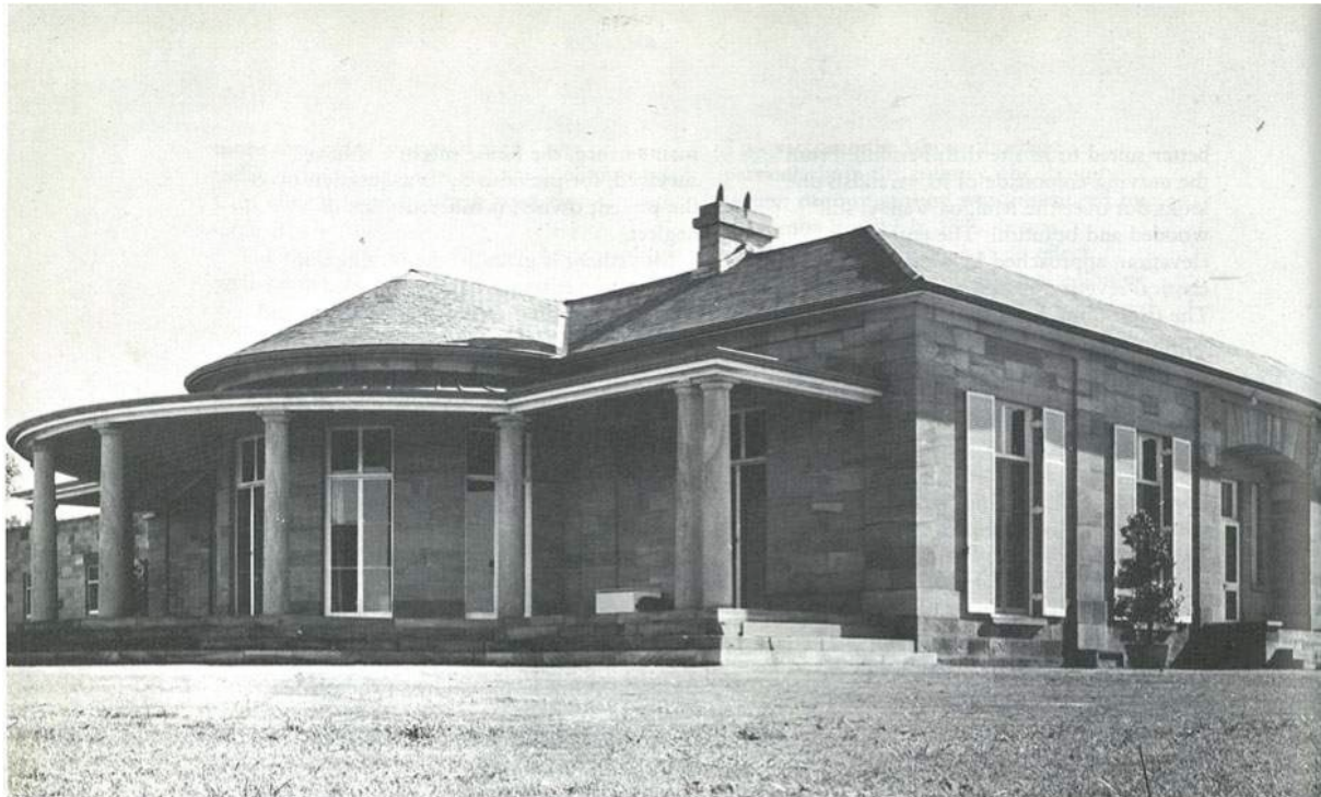
Figure 56: Fernhill, 1975 South Elevation of house showing the porte-cochere removed; Source: Roxburgh 1975:244
