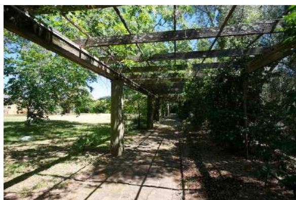
Figure 186: Pergola north of house, looking east. Paul Davies 2014.
