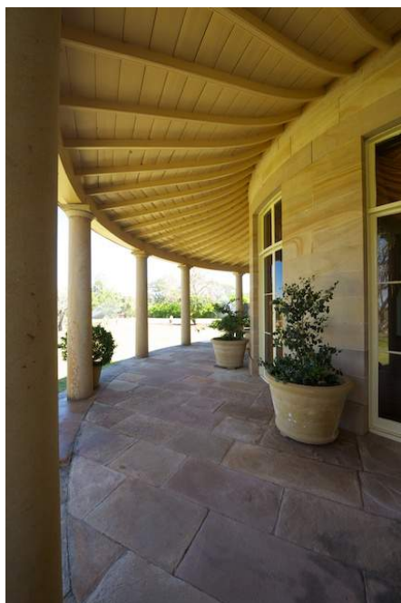
Figure 135: Verandah on southern elevation (G37), looking west. Paul Davies 2013.
