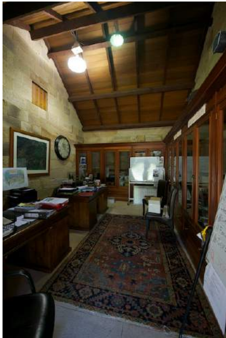
Figure 96: Joinery in central section of stables; new sandstone floor. Paul Davies 2013
