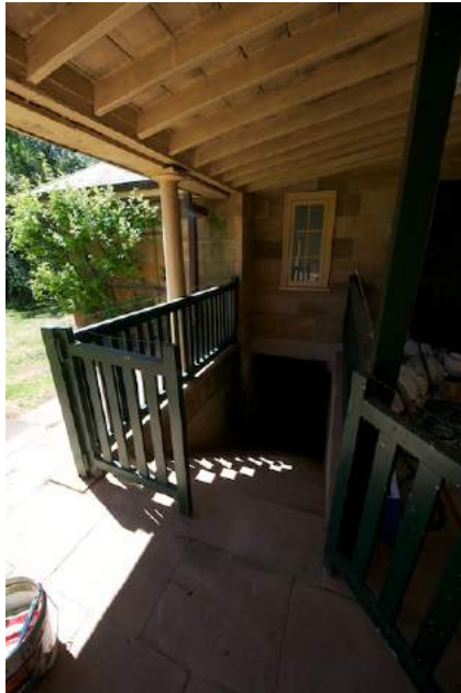
Figure 131: External stair to basement, looking east towards en-suite extension . Paul Davies 2013.
