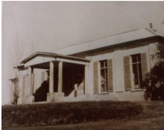
Figure 25: East elevation of house with porte-cochere
