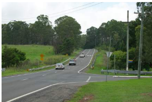
Figure 272: Looking north along Mulgoa Road from the same position as photo 271 was taken showing the nature of the road and the lack of opportunity for pedestrians to stop and traverse the area. Paul Davies 2013.
