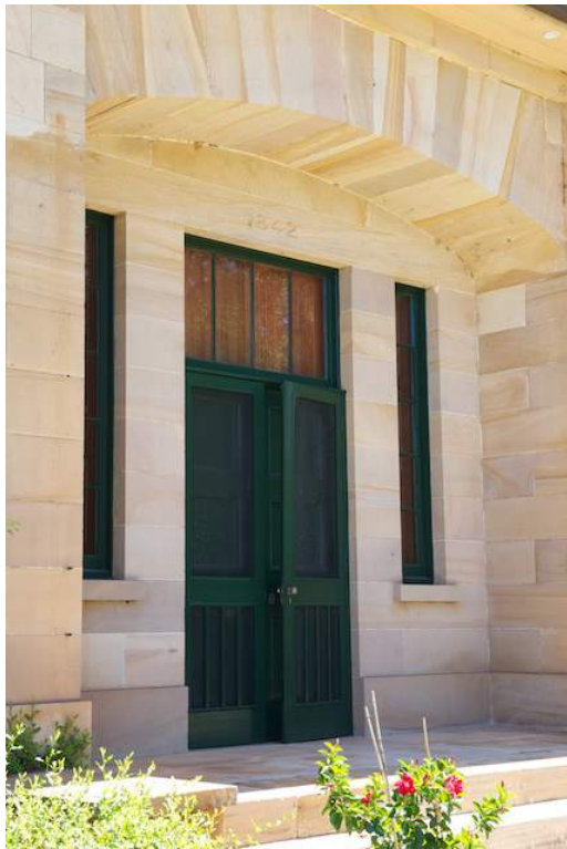
Figure 102: Date of construction above the door lintel, east elevation, 1842. Paul Davies 2013.
