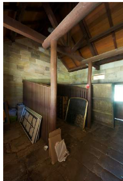
Figure 95: Horse stalls at northern end of stables, looking west. Paul Davies 2013
