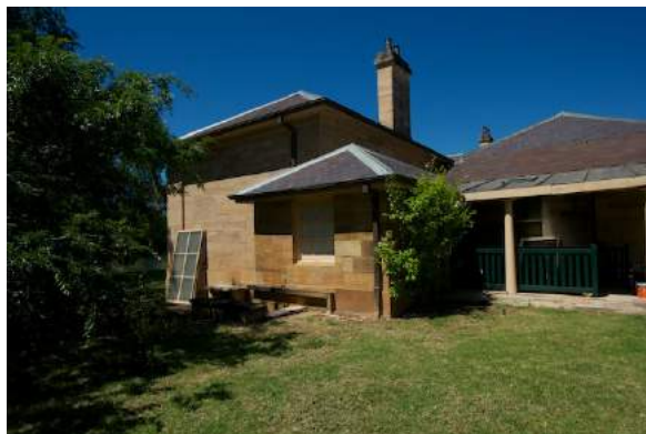
Figure 122: External view of en-suite extension (lower roof) on the north elevation of the house; the taller roof to the left is that of the master bedroom. Paul Davies 2014.
