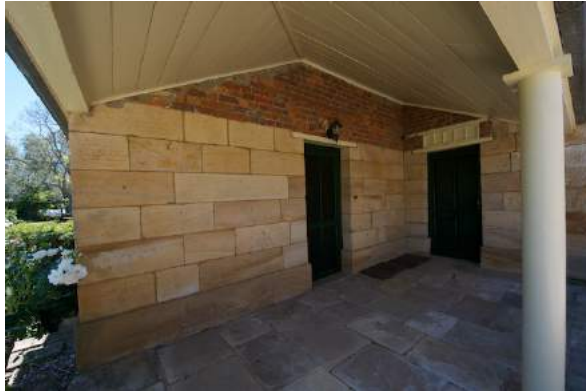
Figure 129: External door to bedroom (G31) with brick courses above sandstone wall to south and west wall under verandah. Paul Davies 2013.
