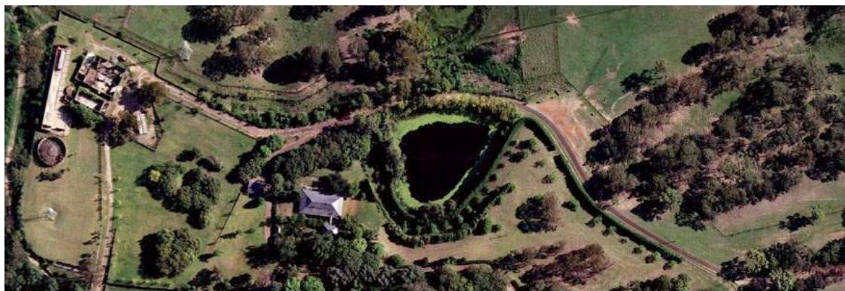
Figure 209: Landscape north of house garden; Manager's Residence; [Source: Google Maps 2010]
