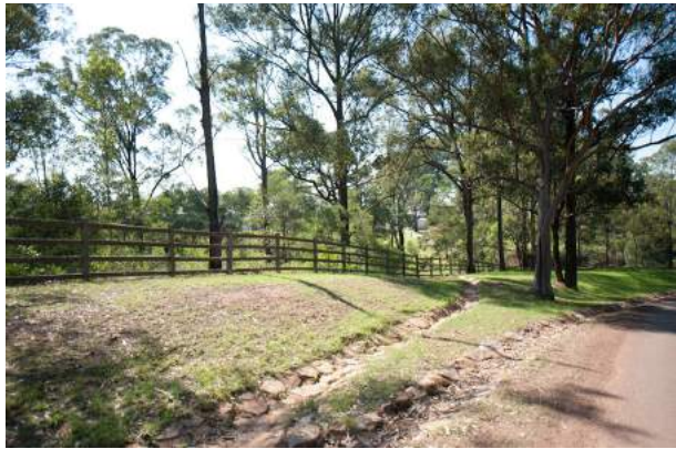
Figure 180: Stone drain along northern side of Southern Driveway in vicinity of original reflecting pond. Paul Davies 2014.
