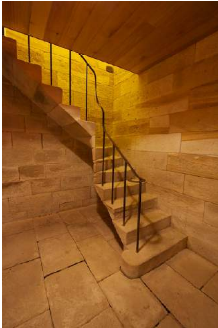
Figure 144: Stone stair from hallway to basement in north wing. Paul Davies 2013.
