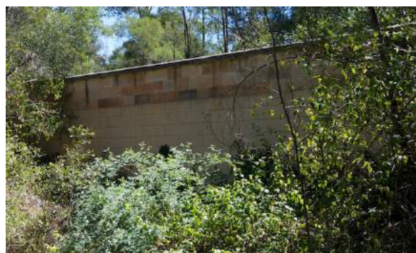
Figure 173: Eastern face of northern bridge, looking west. Paul Davies 2013.
