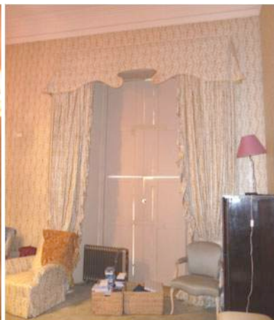
Figure 118: One of the windows on the east wall
