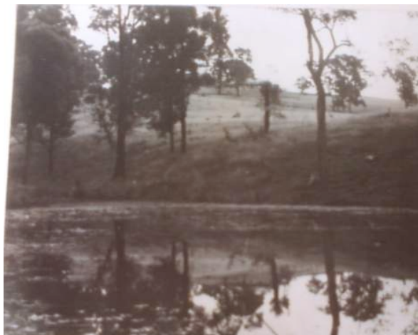
Figure 35: Reflecting pond along driveway showing house (prior to construction of retaining wall and planting of further vegetation in late 20 th century)
