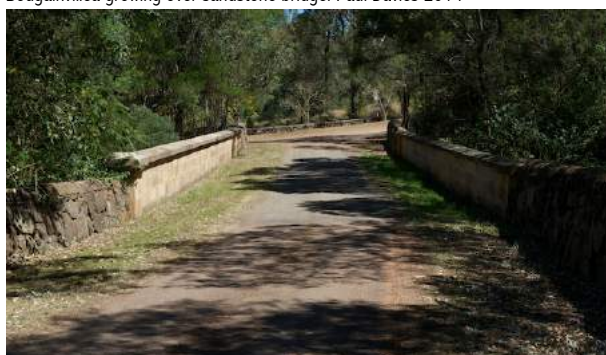
Figure 172: Northern Bridge approach, looking south towards second bridge around bend. Paul Davies 2014.
