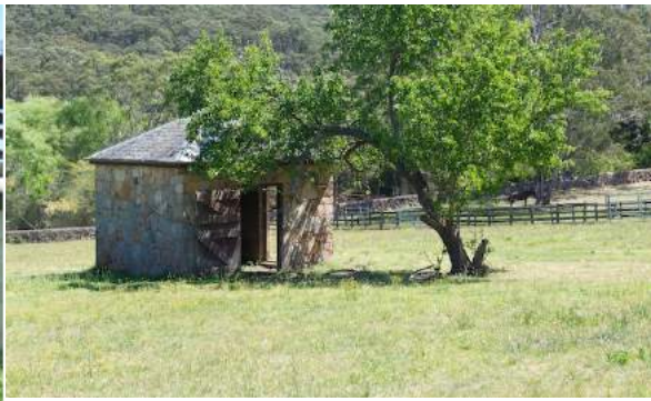
Figure 155: Sandstone loose rubble boxes in paddocks, c. 1980s. Paul Davies 2013
